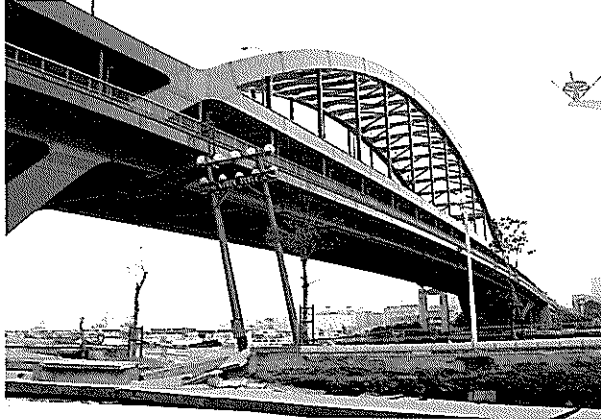
Photo 1 Overview of the Kobe Ohashi Bridge
