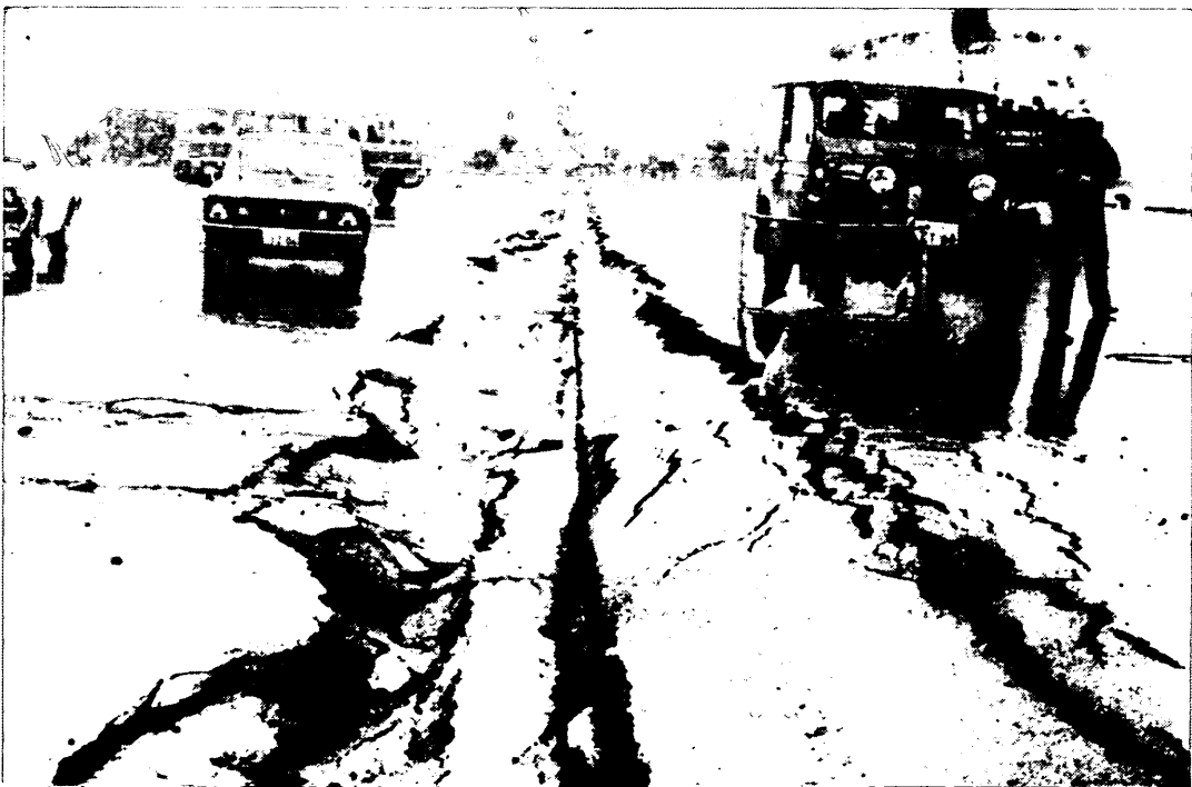
Photo 1 Damages at the quay surface above the anchorage at Nakajima (-10m) Wharf
