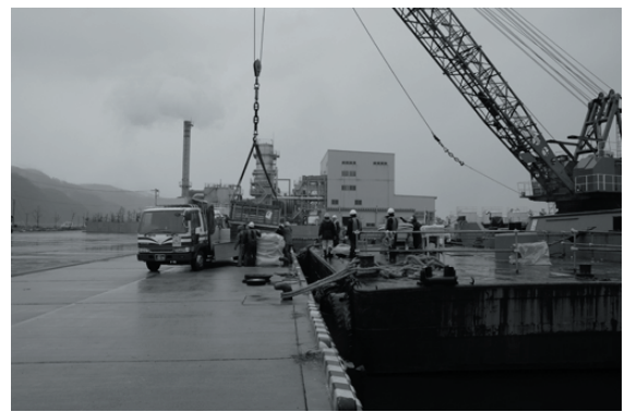
Fig 5. 68 Unloading to the truck bed
