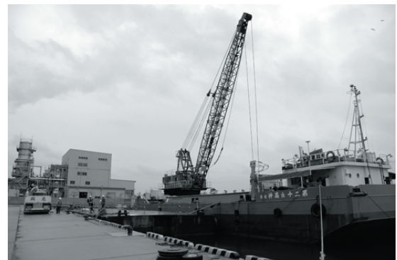
Fig 5. 50 Kojin 26th, crane vessel
