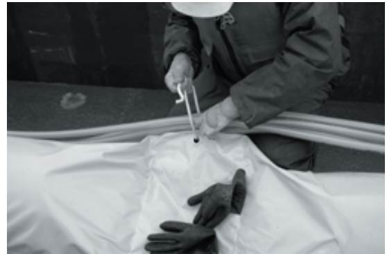
Fig 5.54 Fastening the water jet hose to the boom
