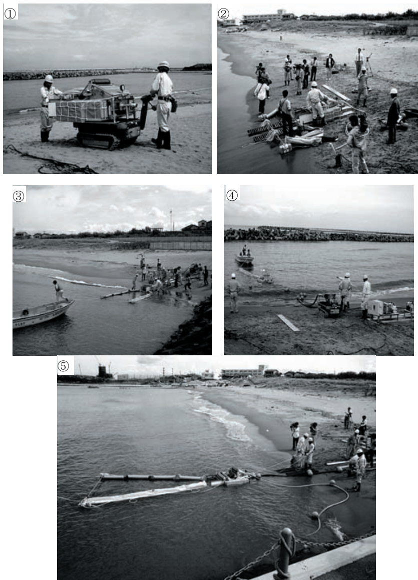
①The crawler carrier ②Preparation of launching ③～⑤Launching
