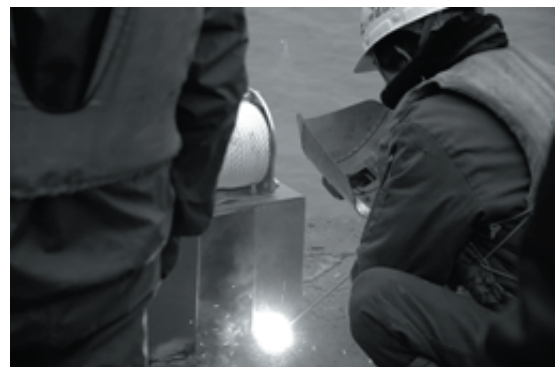
Fig 5.58 Fix the winch on the board (winch tows the buoy)
