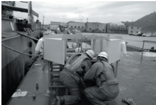
Fig 5.53 Mounting the fixed rudder plate
