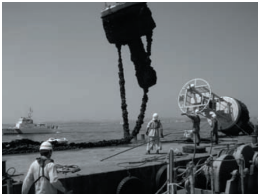
Fig.2.11 Measurement of mooring facility of lighted buoy (Tokyo Bay).
