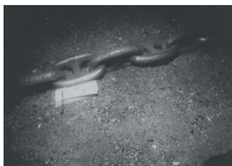
b) Mooring facility of lighted buoy in Tokyo Bay
