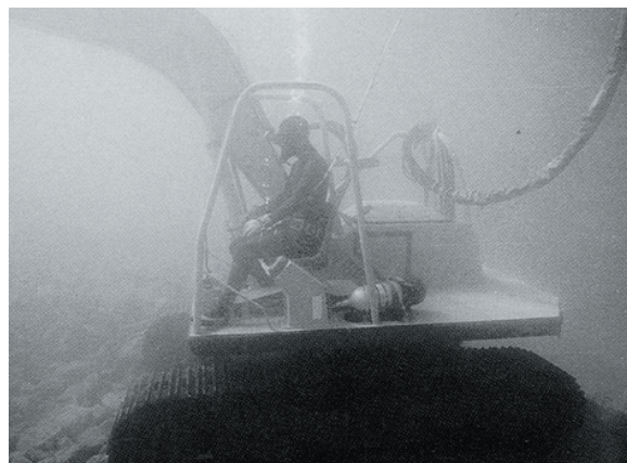
Fig.2.3 Underwater backhoe operated by divers.
