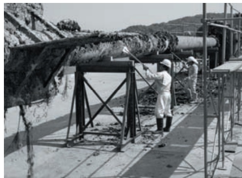
b) Scraping of attached organisms
