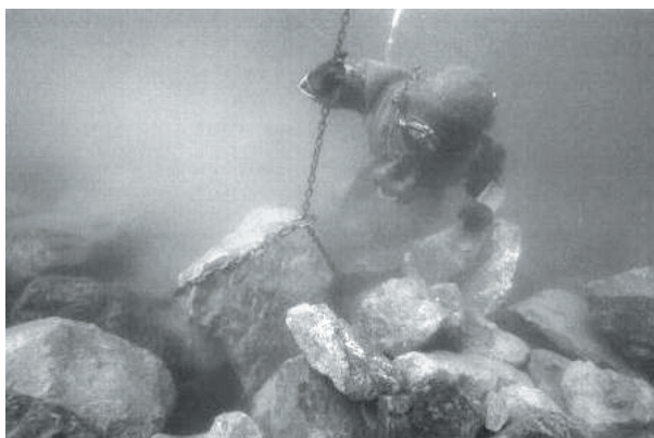
a) Trimming work with crane of vessel
