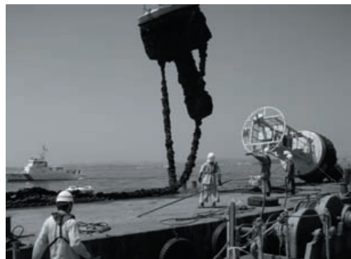
a) Raised buoy on the barge
