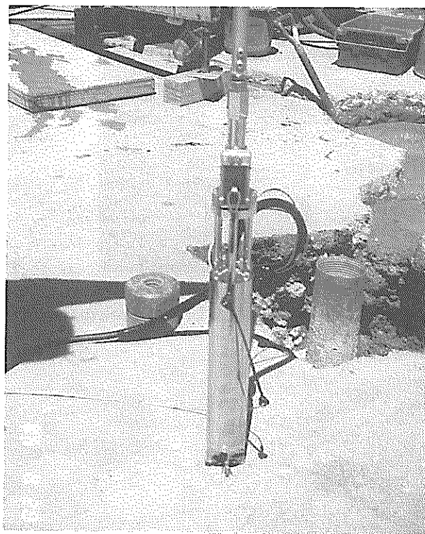
Figure10 Transducers of the ERS-F and -G accelerograph installed in ground
