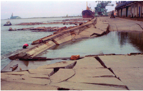
Figure 2. Damage to apron of Gaiko district, Akita port.
