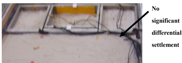
(a) Case A (Sandy backfill) (b) Case B (Backfill with cushion) Figure 24 Ground surface settlements
