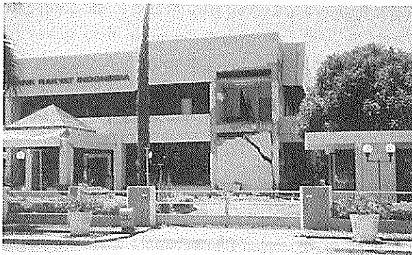
Photograph 1 Damaged bank building in Luwuk (2000)
