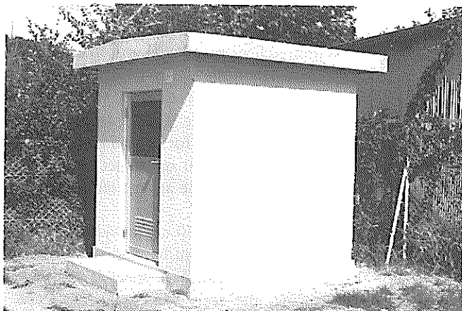
Fig. 22 House of the Onahama-ji-S station
