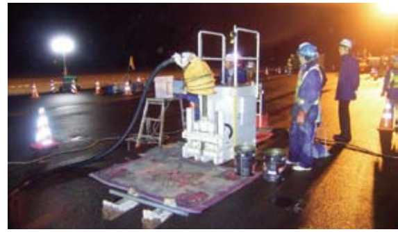
Constructions of a countermeasure against liquefaction at Niigata Airport
