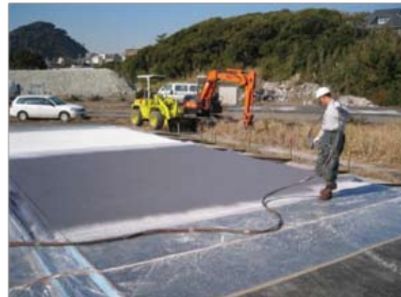
A method to reduce the ground temperature was researched.
