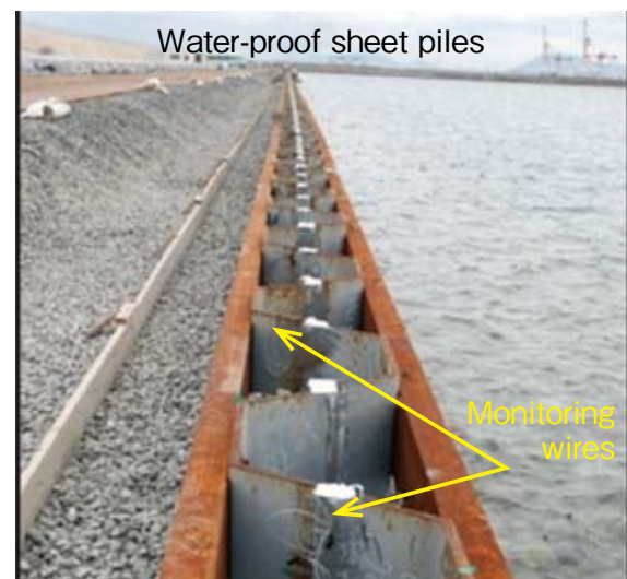
Water-proof quay wall at a waste disposal site in the sea
